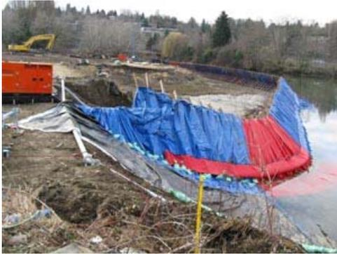
*This February photo shows the "Portadam" used to allow the final excavation of contaminated soils. More photos are available on the website.*
