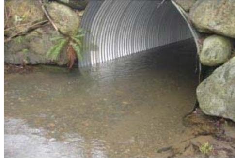
*Culvert showing gravel that has accumulated due to large wood placed downstream. Culvert is no longer a passage barrier.*
