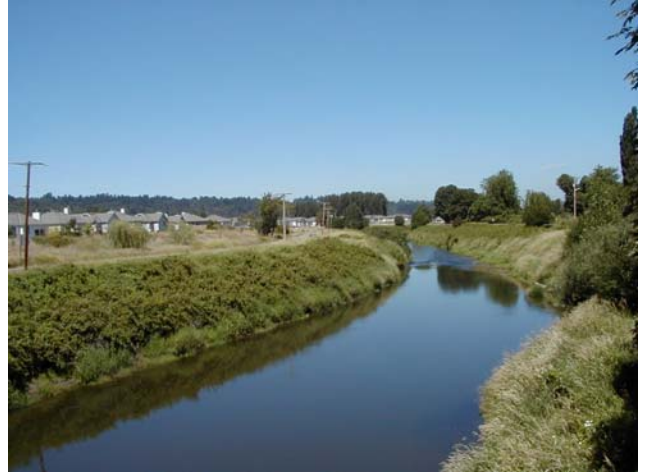
Upstream end of Frager Road Lower project area. Note 200 foot setback of homes on left bank. July 2007 photo.
