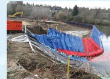
*In February 2009, a "PortaDam" was installed to allow removal of the last contaminated soil on the riverbank.*
