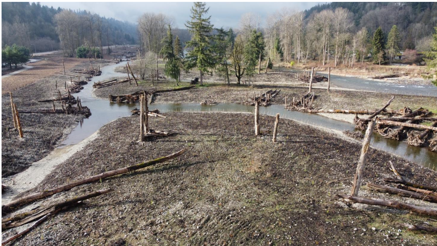
The Riverbend Restoration Project reconnects 52 acres of floodplain habitat and accomplishes 40% of WRIA 8’s goal to reconnect 130 acres of Cedar River floodplain (photo: Seattle Public Utilities).
