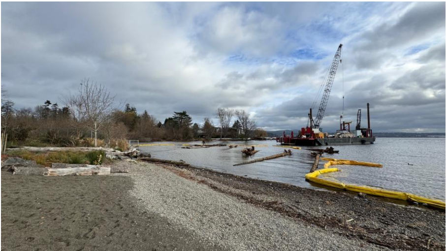
Be’er Sheva Park Shoreline Restoration construction, December 2024.
