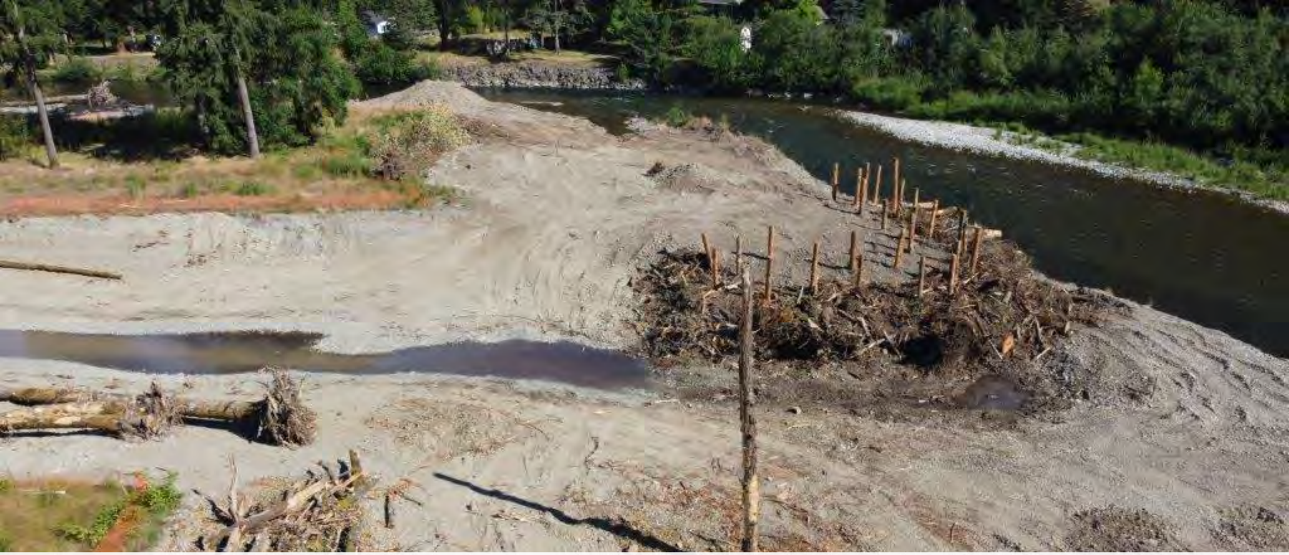
Side Channel and Log Jam Construction
