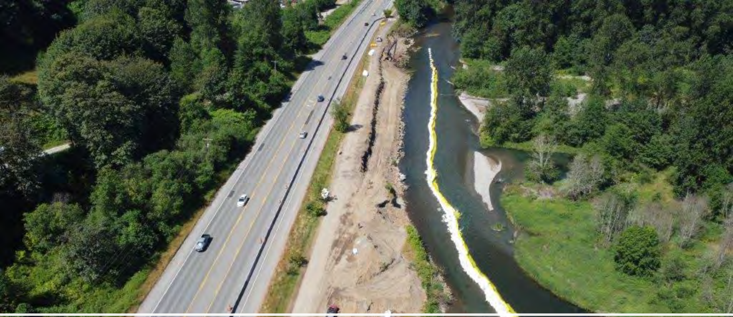
CRT 2 Revetment and Log Jam Construction
