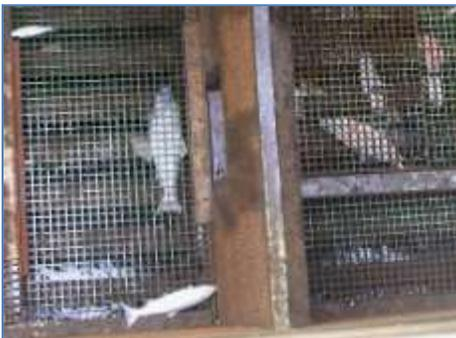
The lower photo shows dead Chinook and sockeye found trapped in the diffuser well underneath the fish ladder. In June 2008, the Corps installed a quick temporary fish screen on the intake. The Corps estimates it would cost \$700,000 to develop alternatives for a permanent solution.
