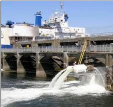
The upper photo shows a ship moving into the large lock, with “smolt passage flumes” in the foreground. The machinery for the gates that open and close the large lock need replacement for continued safe operation and to allow slow opening and closing of the large lock to reduce mortality of juvenile salmon. The flumes provide a safer route for juvenile salmon over the lock spillway. Due to new safety regulations, the Corps must find an alternative to these flumes by spring 2014.
