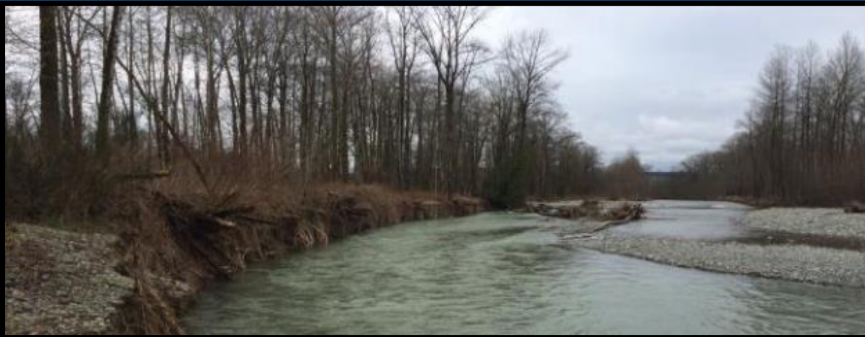
Lower Tolt Project: 2015 after construction
