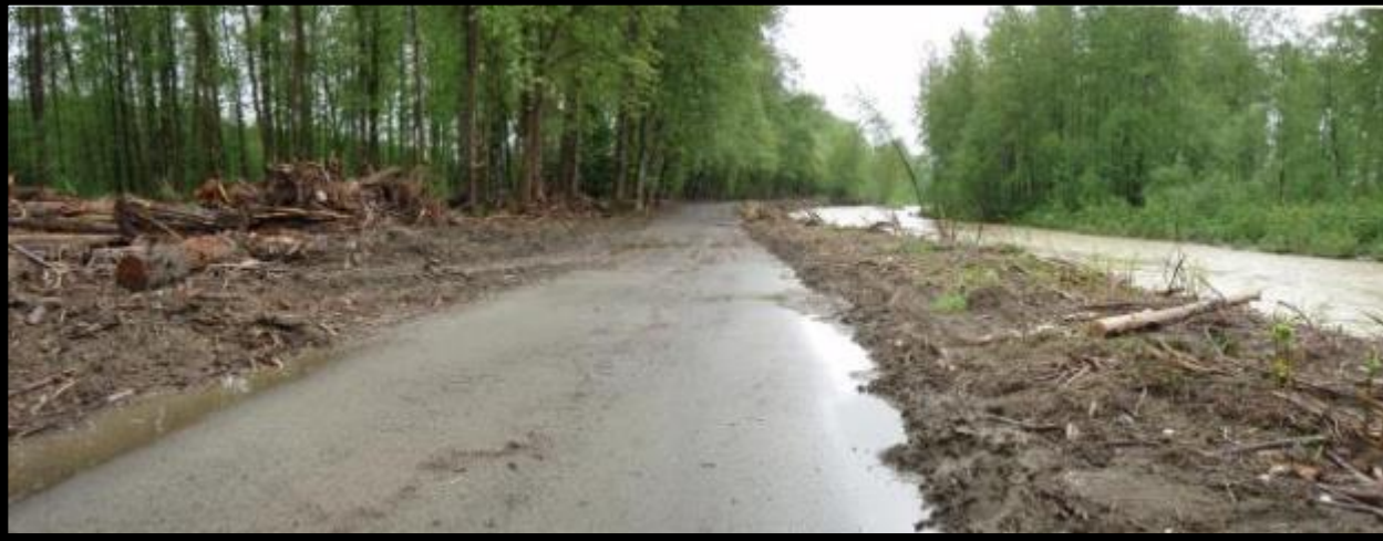
Lower Tolt Project: Before 2009 levee/road removal
