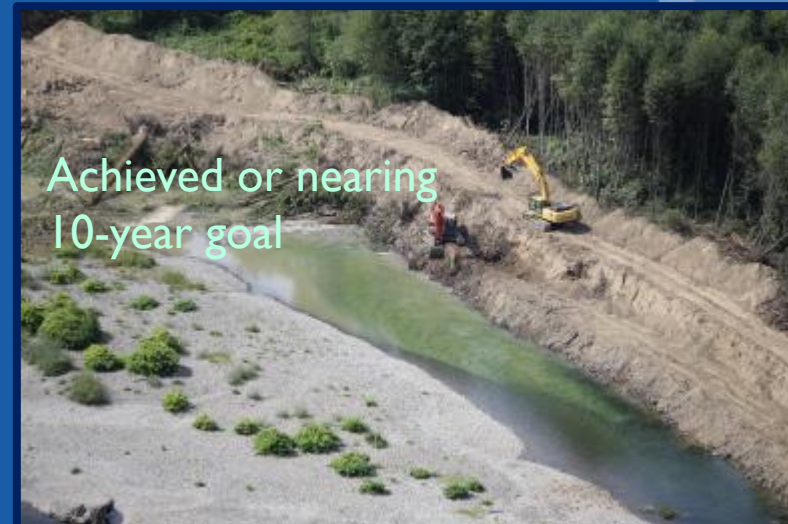
Stillwater Levee Removal Project – Wild Fish Conservancy
