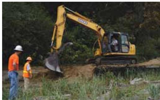
*A decaying, creosote-soaked bulkhead on Piner Point on Maury Island was removed in the summer of 2010. Removal will allow the bluff to erode naturally to feed sediment to the beach.*
