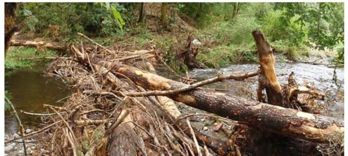
*An engineered log jam installed on Newaukum Creek just upstream of the confluence with the Green River.*
