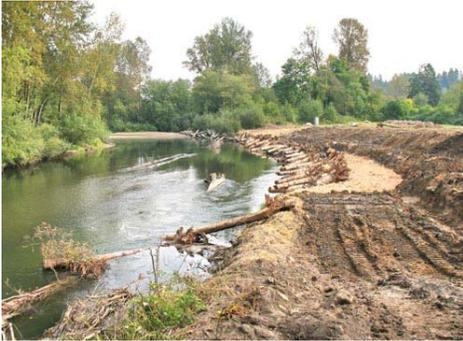
*The Fenster project under construction in October, showing large wood used to armor the toe of the bank.*
