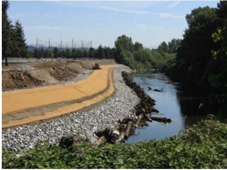
*The Kent Shops-Narita levee on the Green River in Kent while under reconstruction on September 8. Large wood at toe of the levee protects the levee from erosion and provides shelter for juvenile salmon.*
